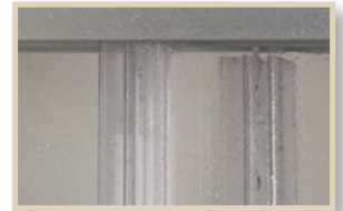
Clear weatherstripping mounts on overlapped doors.
